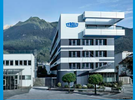
Tyrolit headquarters in Schwaz (Austria)
